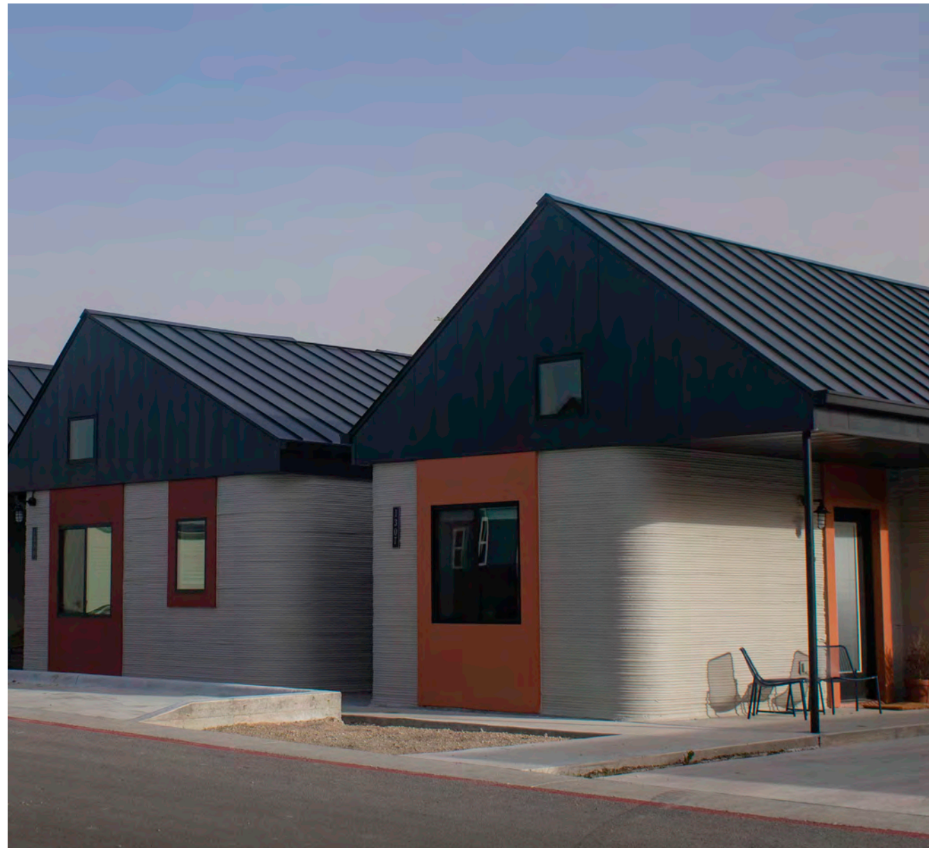
HOUSES BUILT USING 3D PRINTED CONCRETE
